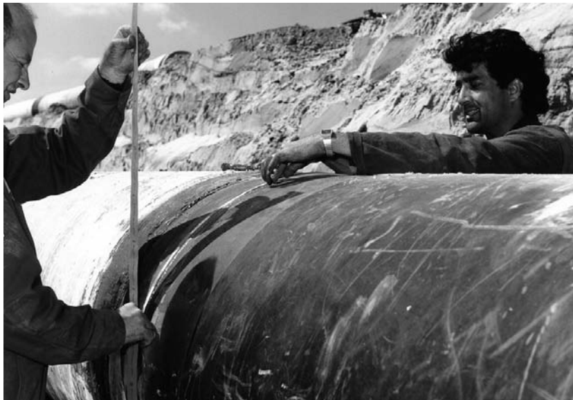
Fig. 14-18. Preparation of strip film on girth weld
