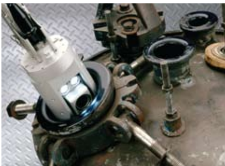
Inspection through a 100mm (3.94 in) \emptyset nozzle
